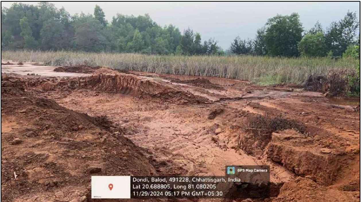
Tailing storage pond inside the unit
